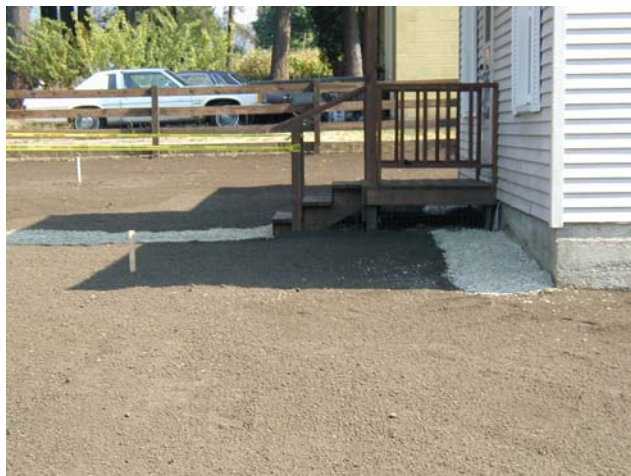
Property undergoing remediation
