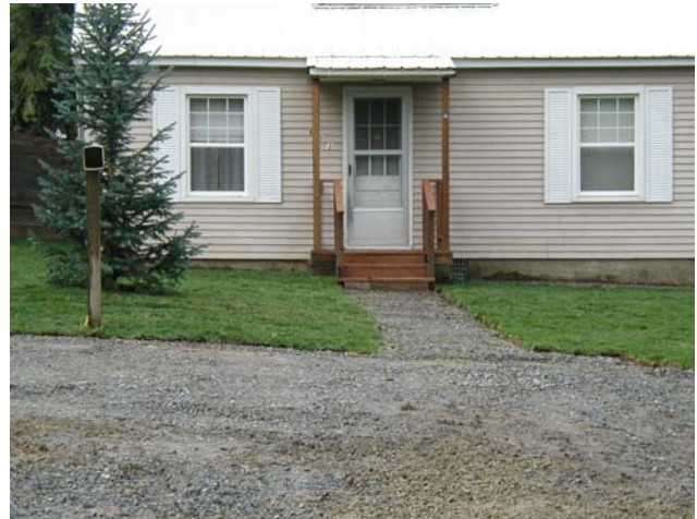
Property after remediation
