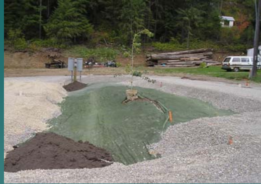
Contaminated soils removed, protective barrier placed, backfill in process.
