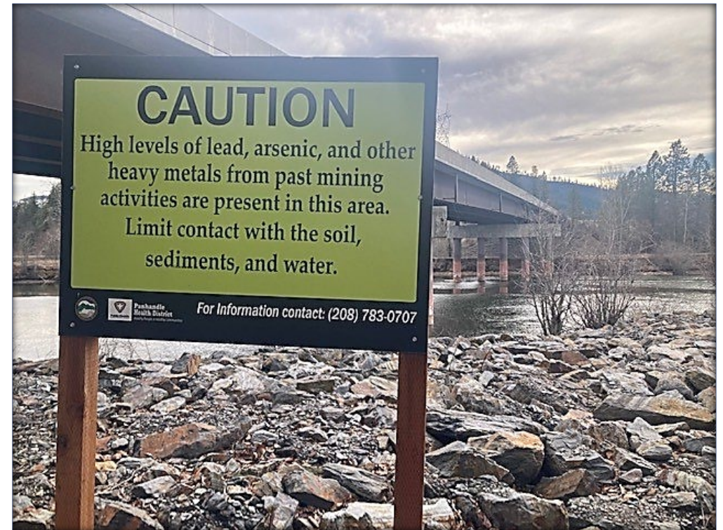
Hwy 3 bridge remediation complete : Photo courtesy of BEIPC
