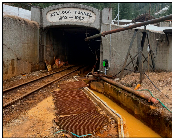
Figure 3. Acidic and metal-rich mine water discharging (channel along the cement berm) from the Bunker Hill Mine portal (Kellogg Tunnel).
