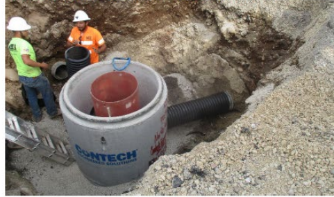
CDS Structure install
