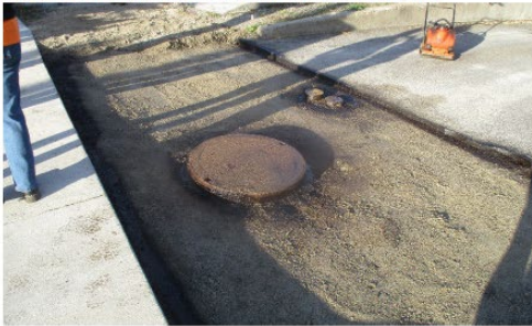
Prepped for asphalt installation
