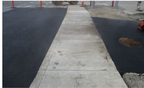
Complete repaired area around CDS structure
