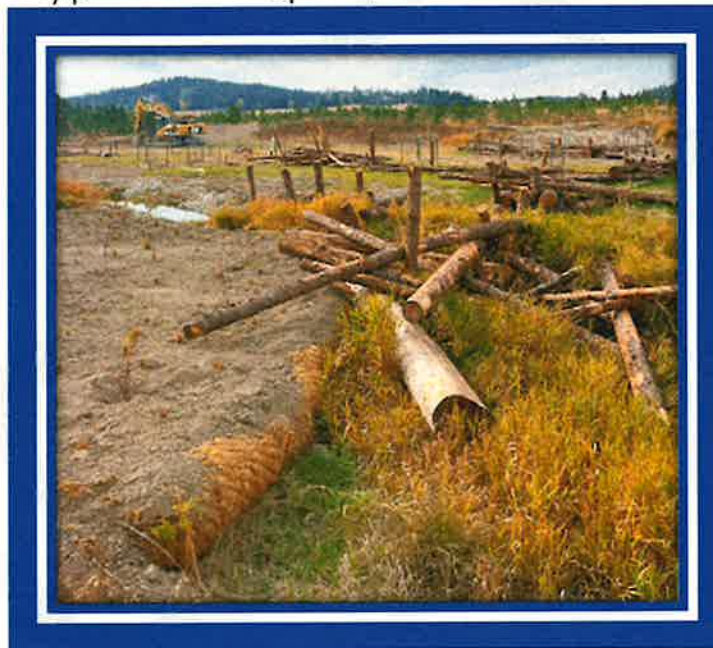
In-channel and floodplain placements of large wood on upper Lake Creek. Photos courtesy of RP.
