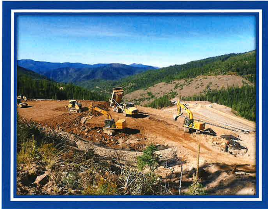
East Fork Ninemile Waste Consolidation Area waste placement. Image provided by the CDA Trust.
