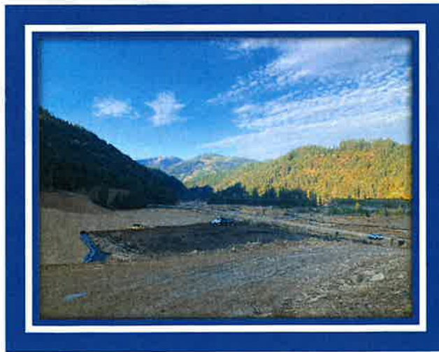
Canyon Creek Repository. Picture provided by EPA.
