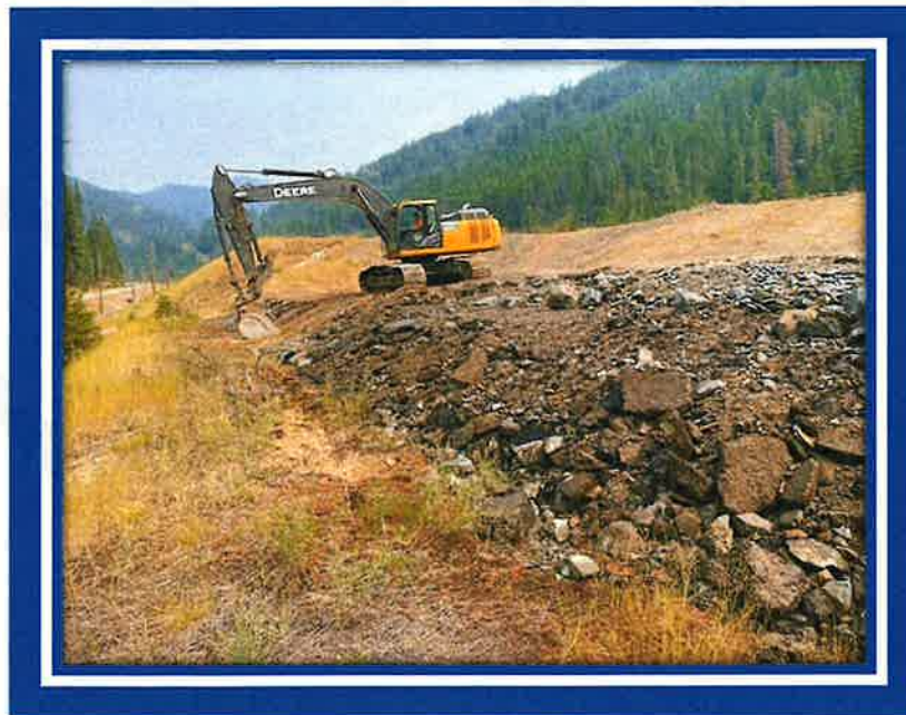
Lower Burke Canyon Repository waste grading. Image provided by the CDA Trust.
