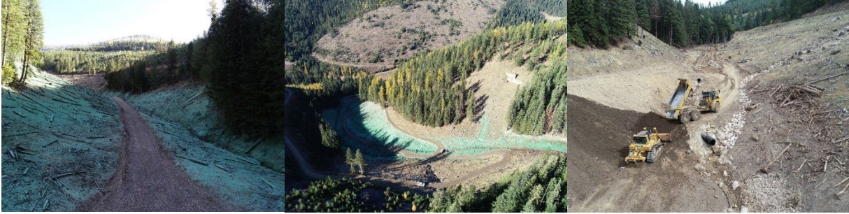
Tamarack remediation and reconstruction. Provided by the CDA Trust.
