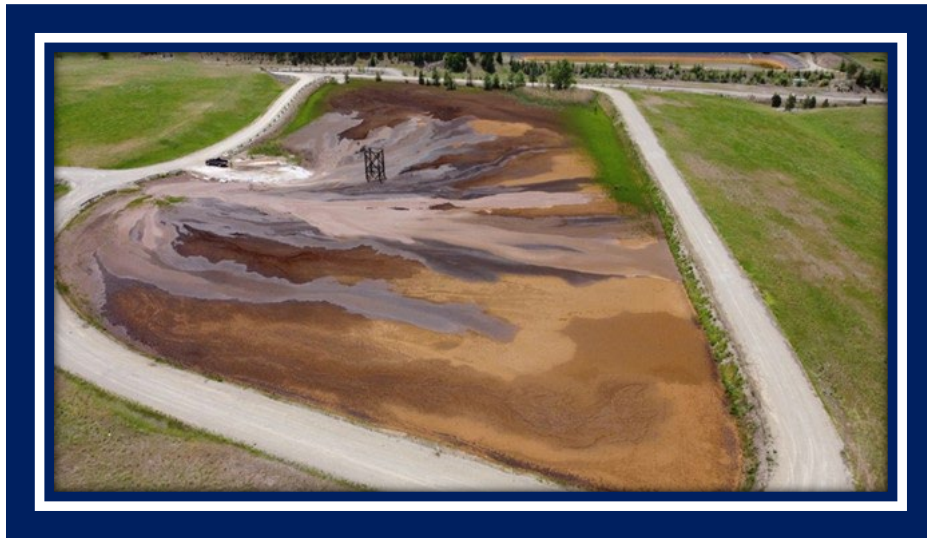
Old Sludge Pond looking south. Photo courtesy of USACE Seattle District.
