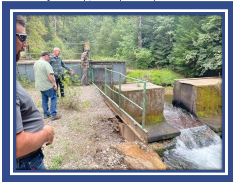
Big Creek fish barrier. Photo courtesy of RP.
