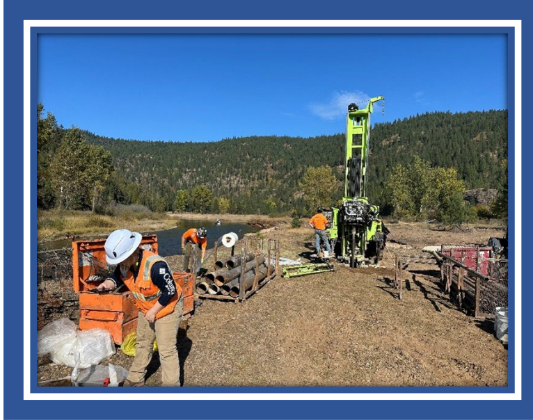
Cataldo Riverbank Pilot Project. Photo courtesy of CDA Trust.
