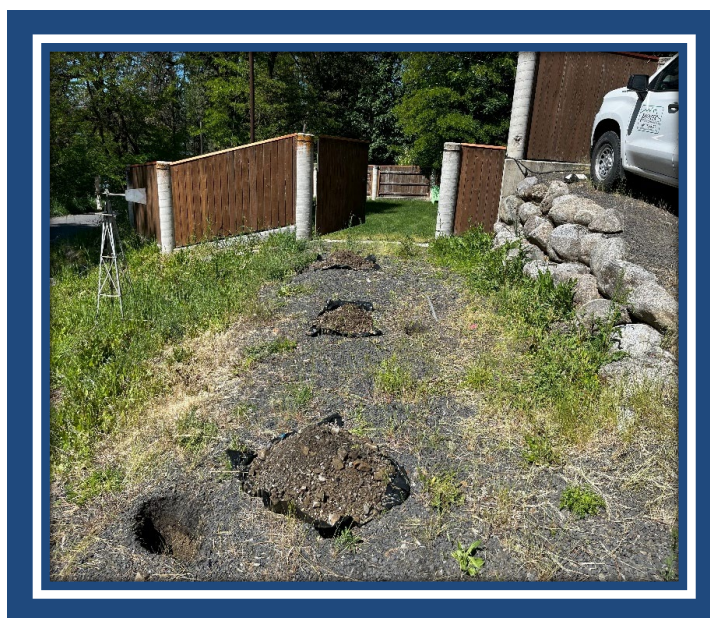
Looking West. Completion of soil sampling. Image provided by CDA Trust.
