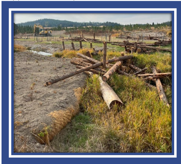
In-channel and floodplain placements of large wood on upper Lake Creek. Photos courtesy of RP.
